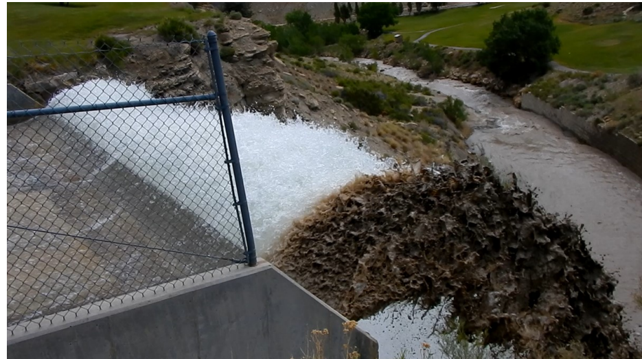
Figure 1. Millsite Lake—An Example of a Reservoir that Passes Dredged Sediment to the Downstream Channel
