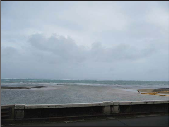
Photo 2. November 30, 2009 looking east and seaward from bridge.
