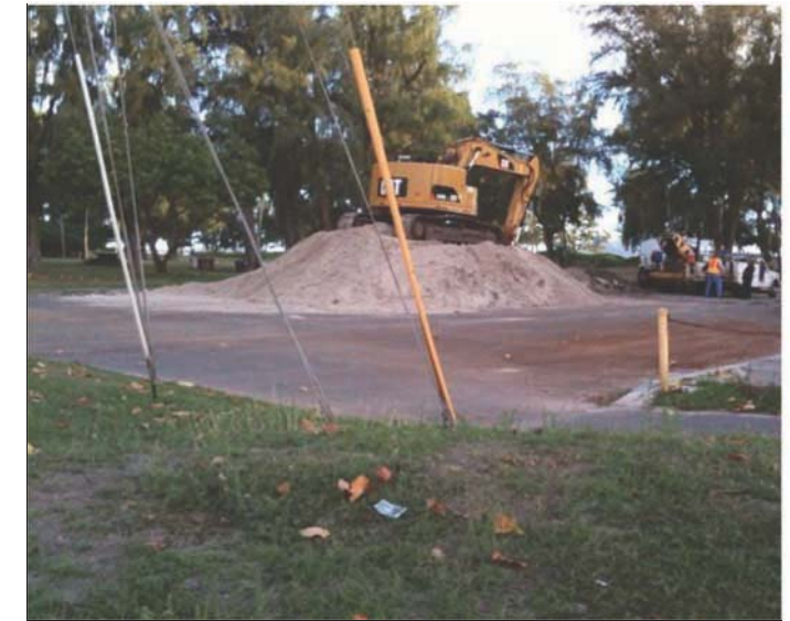
Photo 2. October 19, 2009 sand from stream mouth clearing.
