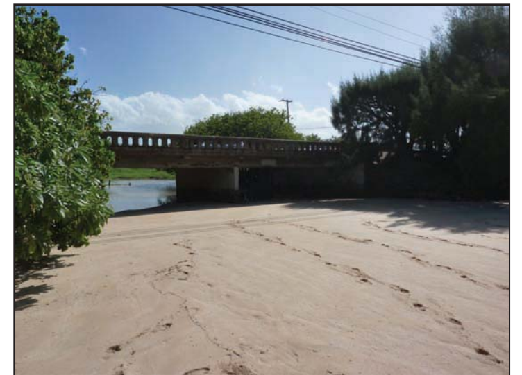
Photo 2. December 5, 2009 looking landward at the bridge from Laniakea Beach.
