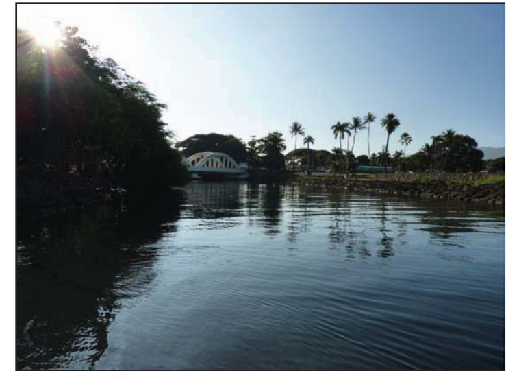
Photo 2. December 14, 2009 looking upstream toward the bridge and Haleiwa.
