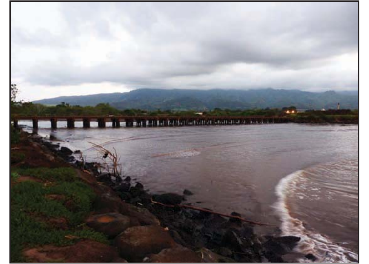
Photo 2. December 13, 2009 looking landward and at the bridge in Kaiaka Bay.
