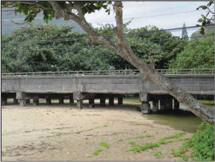
Photo 2. November 30, 2009 looking landward and south back under the bridge.
