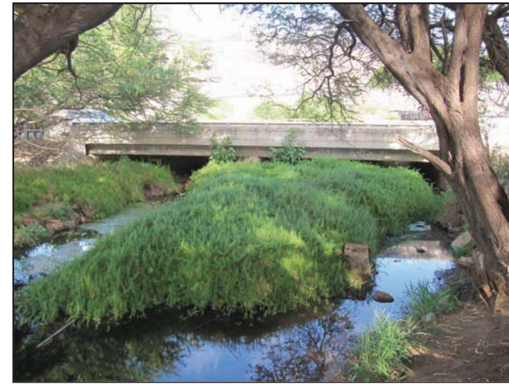
Photo 1. November 30, 2009 looking landward toward the Kahe Stream Bridge.
