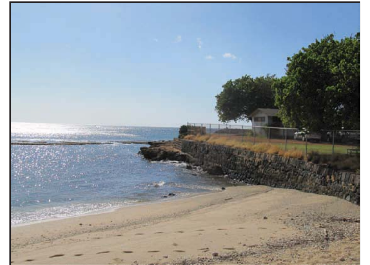
Photo 2. November 29, 2009 looking at the beach and seawall directly north of the stream mouth.
