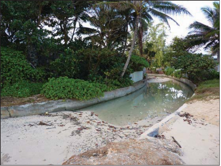
Photo 2. November 30, 2009 looking seaward, down stream from the bridge.
