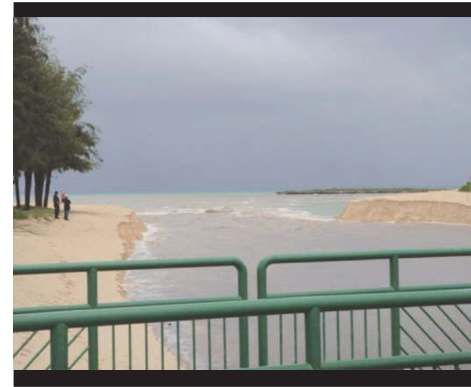
Photo 1. October 19, 2009 looking down stream from the bridge to the stream mouth.
