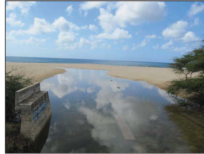
Photo 1. October 24, 2009 looking seaward from the road.
