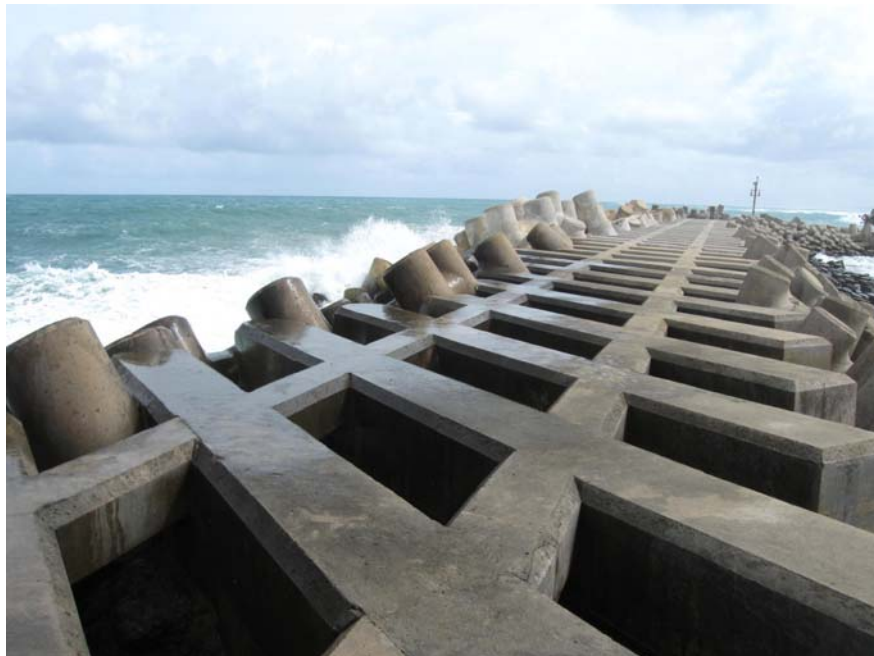
a. Sta. 20+87 , no damages noted.
