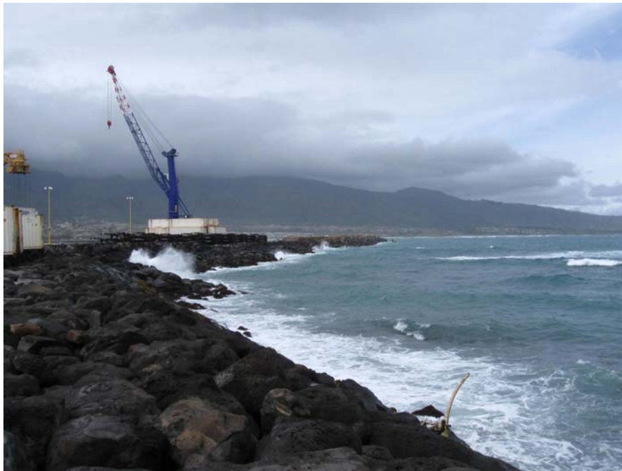
Overview of breakwater at Sta. 8+00, no changes noted.
