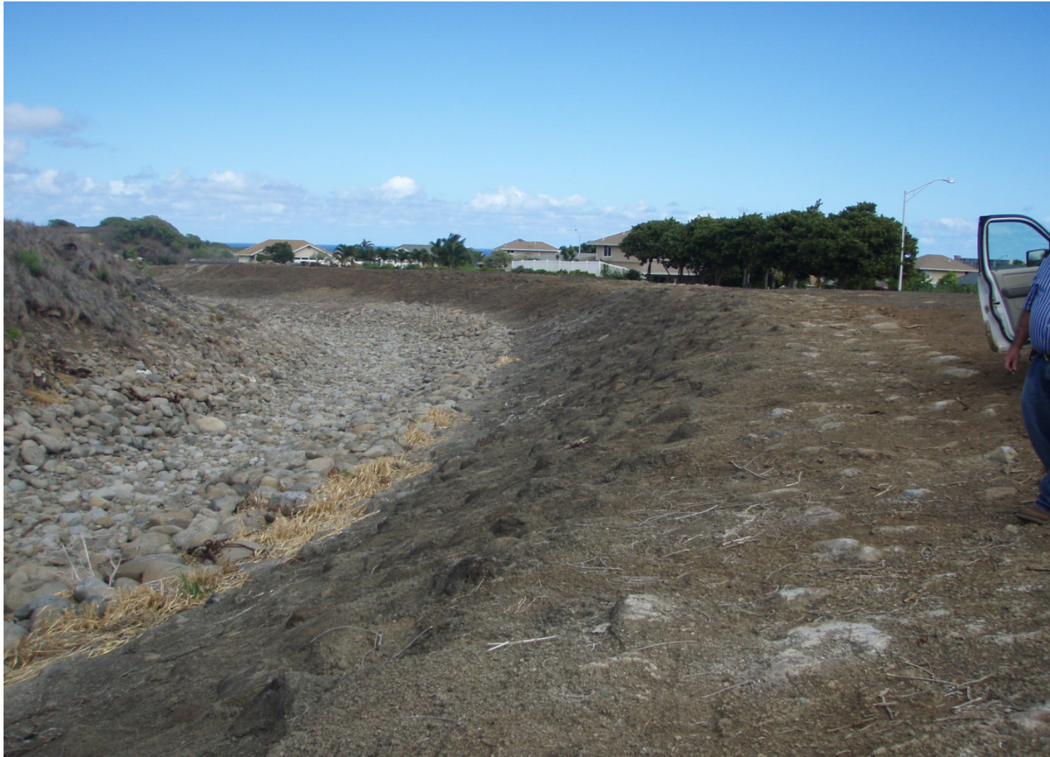
Inspect ID: ISLE_2009_a_0003 Name: Levee Embankment Caption: Sta. 67+00, ( Levee D) Unwanted vegetation removed, sideslope and natural chnl being maintained
