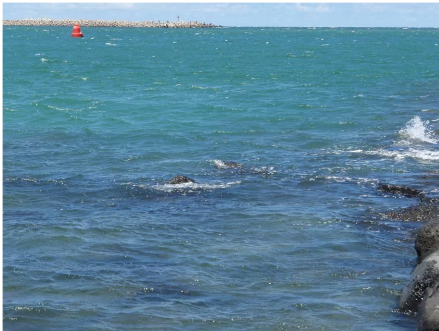
c. Sta. 1+50, Centerline Crest (CL), Scattered stones are remnants of the old LST landing site. No changes this year.
