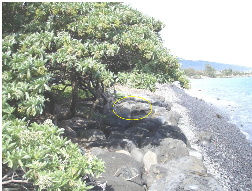
i. Sta. 8+90, Monitor settling at crest. No additional settling this inspection.
