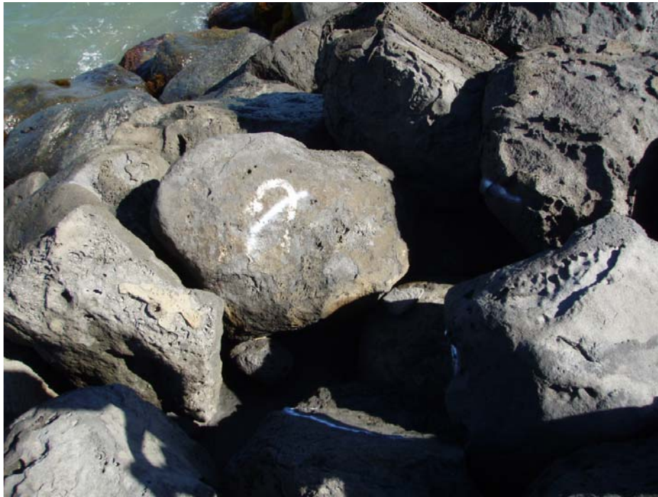
c. Sta. 12+00, Reset armor stone in 2 ft. void on sideslope.
