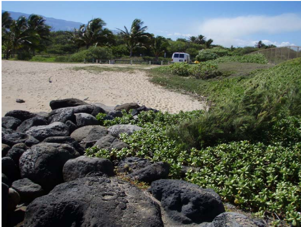
n. Sta. 15+90, Overview, remove vegetation from armor stones..
