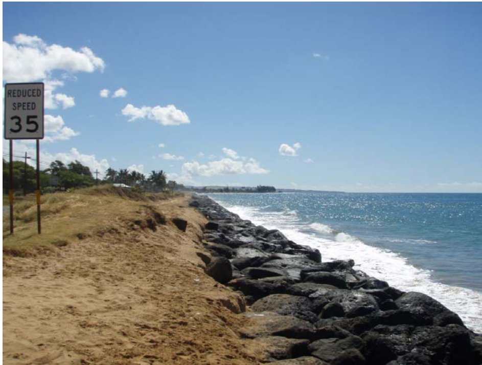
e. Sta. 11+85, Overview, monitor armor stones post storm event.
