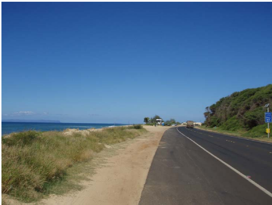
d. Sta. 11+50, Overview, cut grasses, Reference Call Box # 506269.
