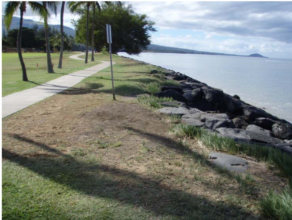
b. Sta. 2+90, Fill material added to eroded area.
