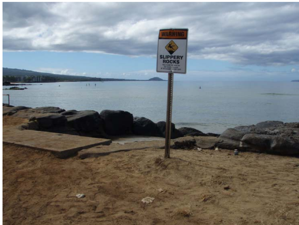
u. Sta. 23+50, Access walkway with recent repairs.
