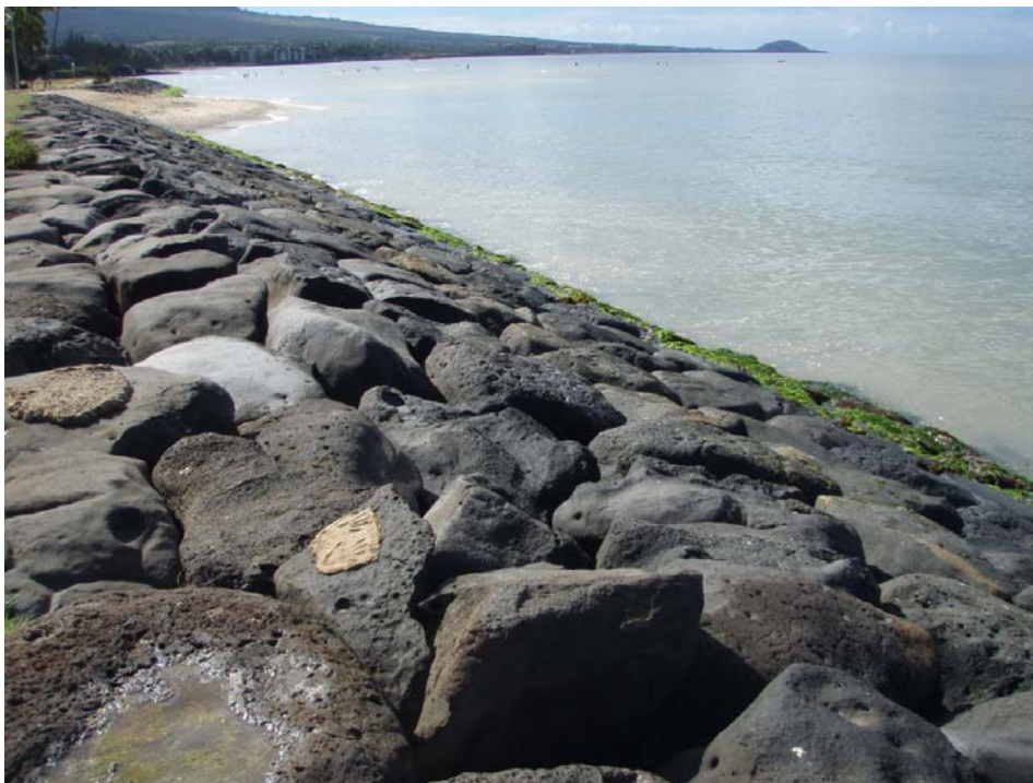
k. Sta. 10+00, Monitor settling on sideslope, no change this year.
