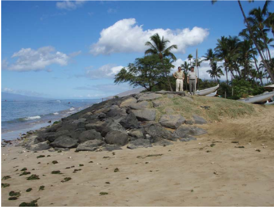
x. Sta. 26+97, End of project (south), reference photo.
