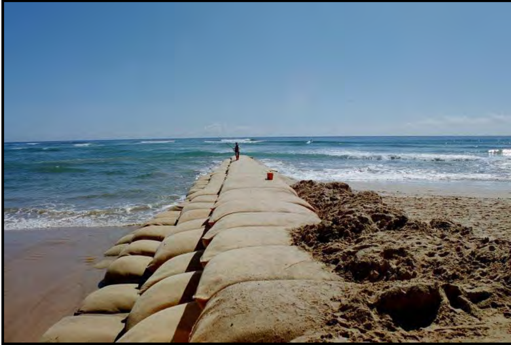
Figure 5-14 ELCORock Groin, Maroochydore, Australia (source: Geofabrics Australasia)
