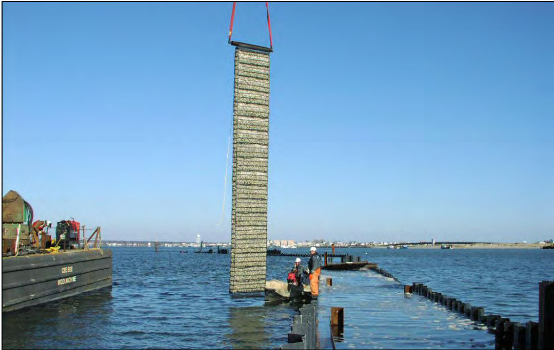
Figure 5-29 Deployment of Triton Marine Mattress (source: Tensar International)
