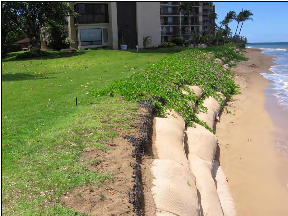
Figure 5-25 Hololani shore protection, August 25, 2008 (Sea Engineering photo)
