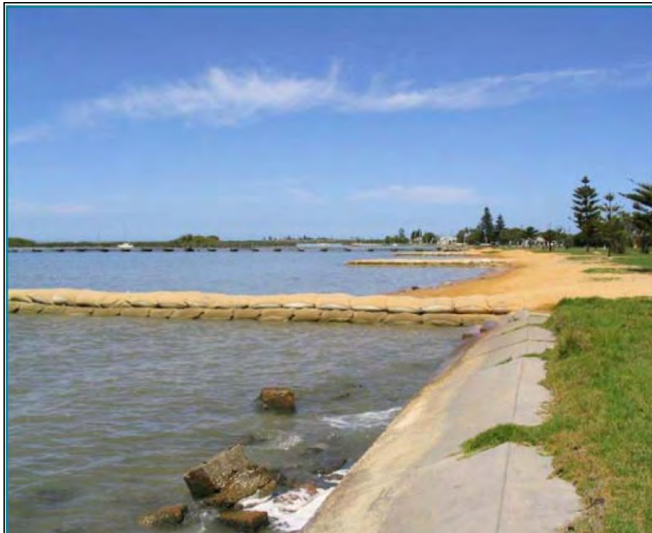
Figure 5-15 Milang, Australia, shore protection, old (foreground) and new (background); (source: ELCO Solutions)
