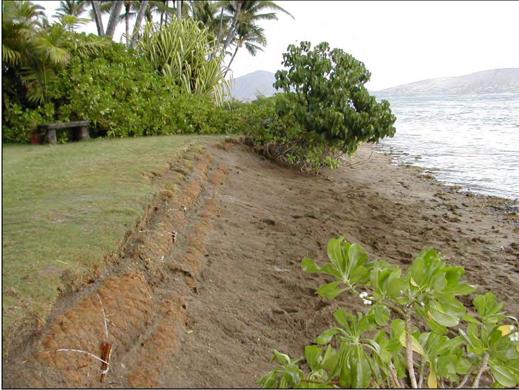
Figure 5-35 Coir logs stabilizing the vegetation line at an East Oahu location
