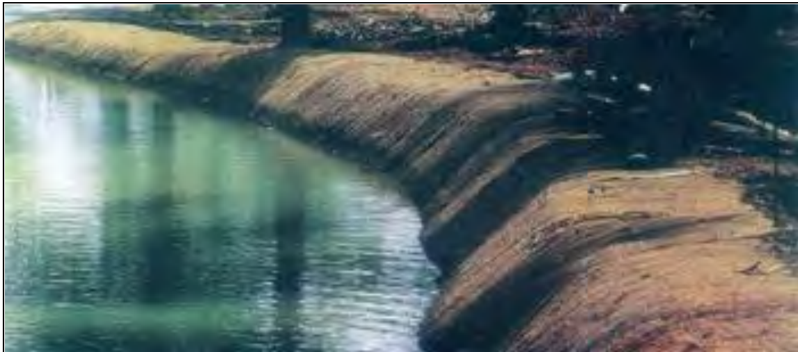
Figure 5-34 Stream bank protection using coir geotextile (source: www.unitedcoir.com )
