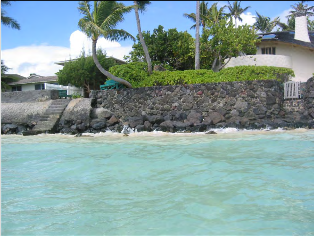
Figure 6-5 Photo of shoreline at termination of south groin
