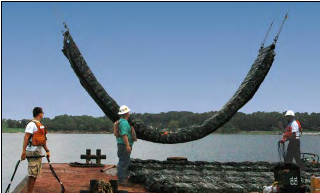
Figure 5-30 Deployment of a Triton Marine Mattress (source: Tensar International)
