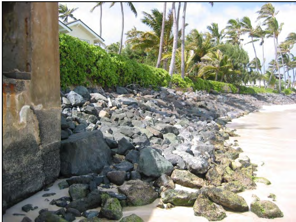
Figure 2-6 Rock revetment to the north of the seawalls
