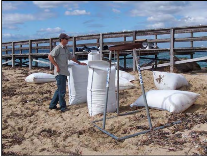
Figure 5-10 Filling procedure for a 0.35 m 3 ELCORock Bag (source: Geofabrics Australasia)
