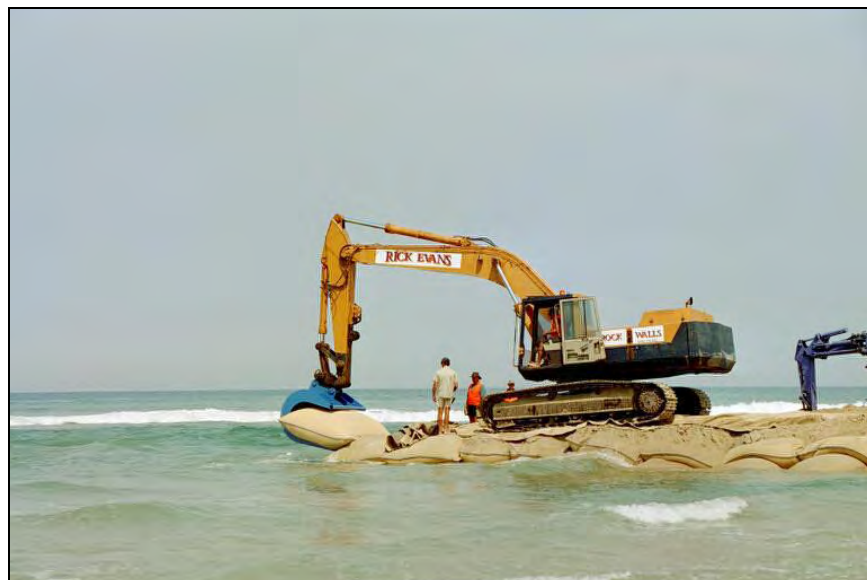
Figure 5-18 Placing of bag
