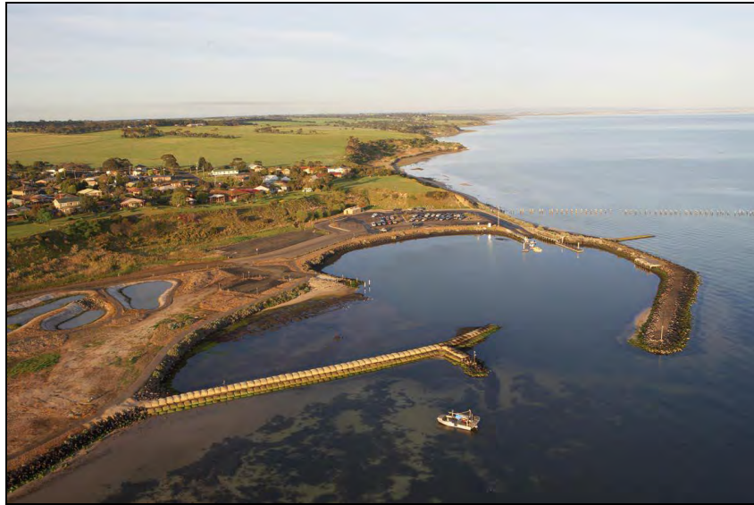
Figure 5-16 ELCORock groin, Clifton Springs, Australia (source: ELCO Solutions)
