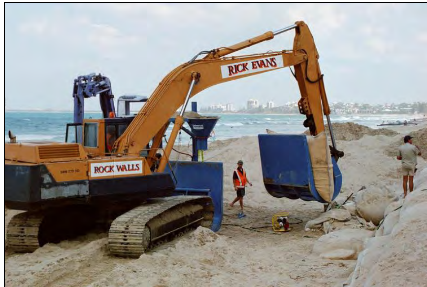
Figure 5-17 Excavator carrying a 2.5 m 3 ELCORock bag
