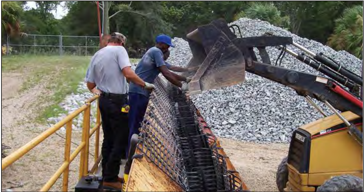
Figure 5-27 Workers filling a Triton Marine Mattress (source: Tensar International)
