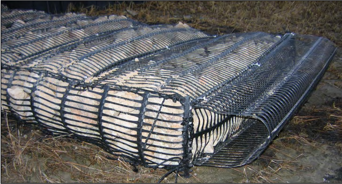
Figure 5-21 View of Triton Marine Mattress (source: US Army Corps of Engineers)
