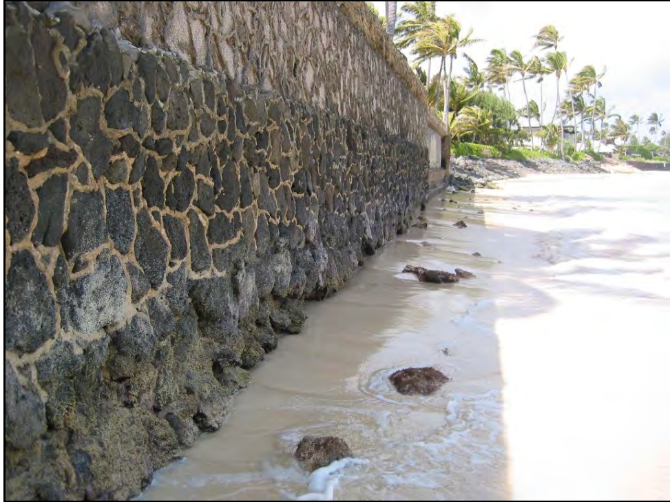
Figure 2-5 Vertical seawalls on north side of beach access
