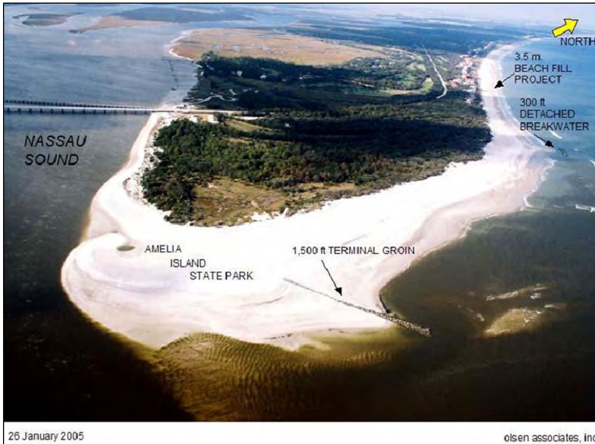
Figure 5-23 Amelia Island Shoreline Restoration, post construction (source: US Army Corps of Engineers)
