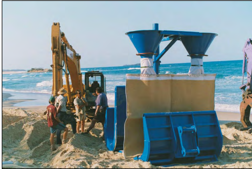
Figure 5-12 Assembled apparatus on site
