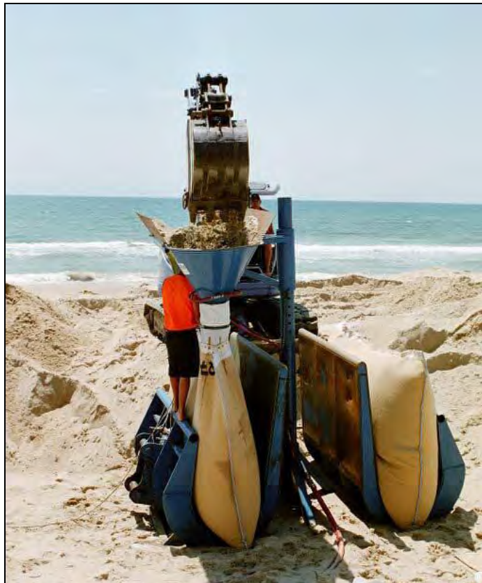
Figure 5-13 Filling of 2.5 m 3 bags
