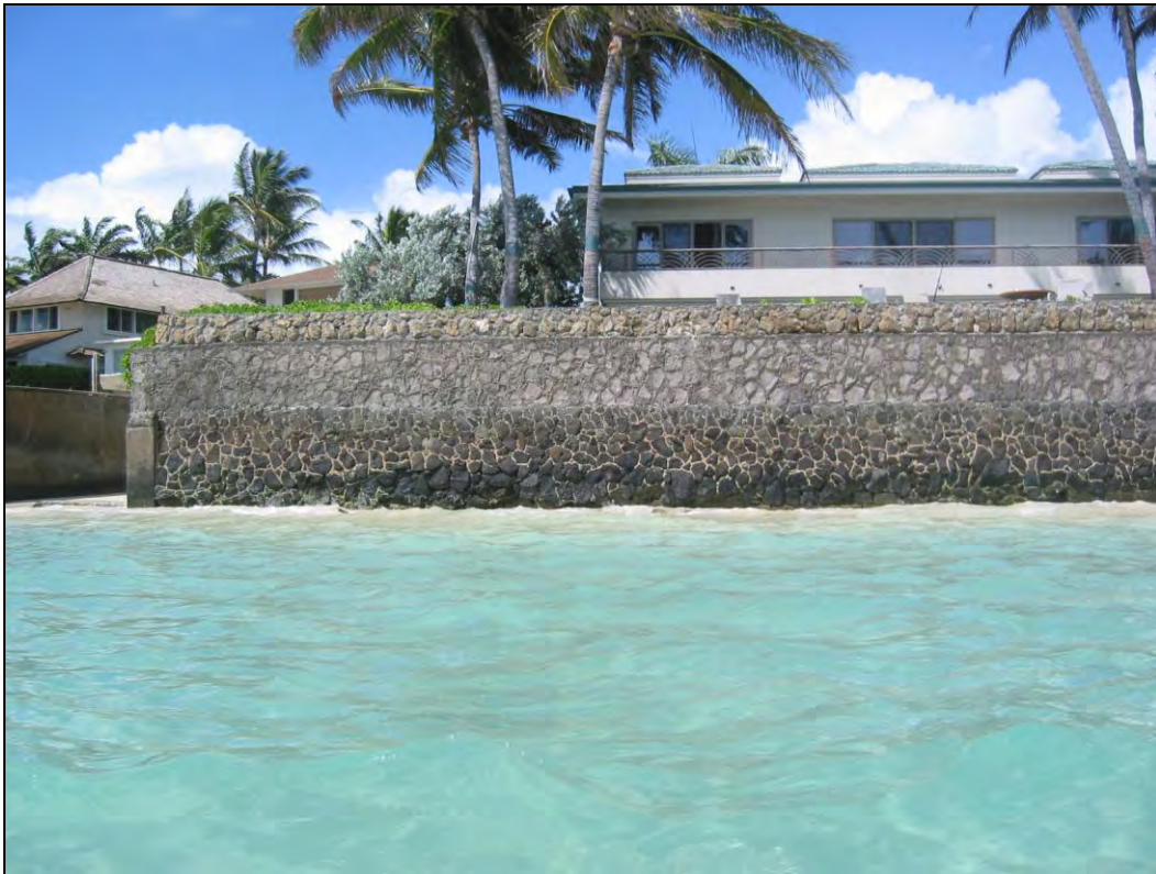
Figure 6-6 Photo of shoreline at termination of north groin
