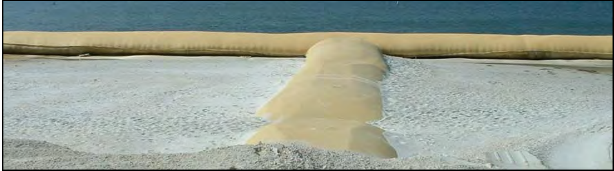
Figure 5-1 Oblique view of T-groin constructed of MacTubes (source: Maccaferri USA)
