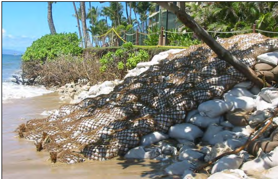
Figure 5-37 Coir and sand bag revetment in place
