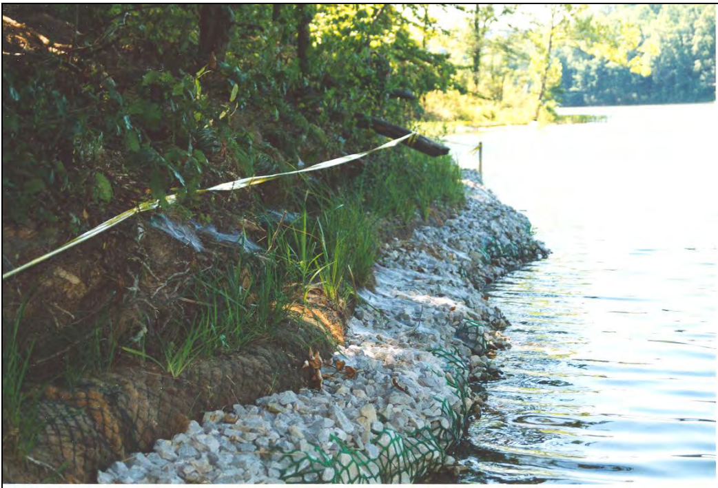
Figure 5-36 Coir log stabilizing bank (source: Geotech Solutions Hawaii)
