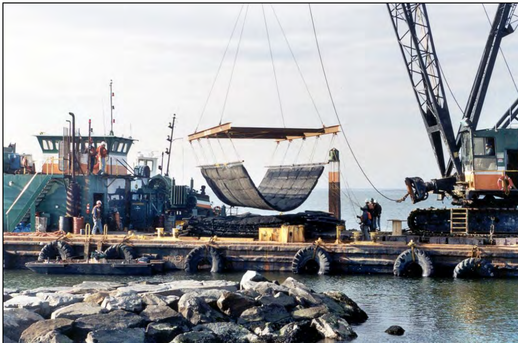
Figure 5-28 Deployment of Triton Marine Mattress—three units wide (source: Tensar International)
