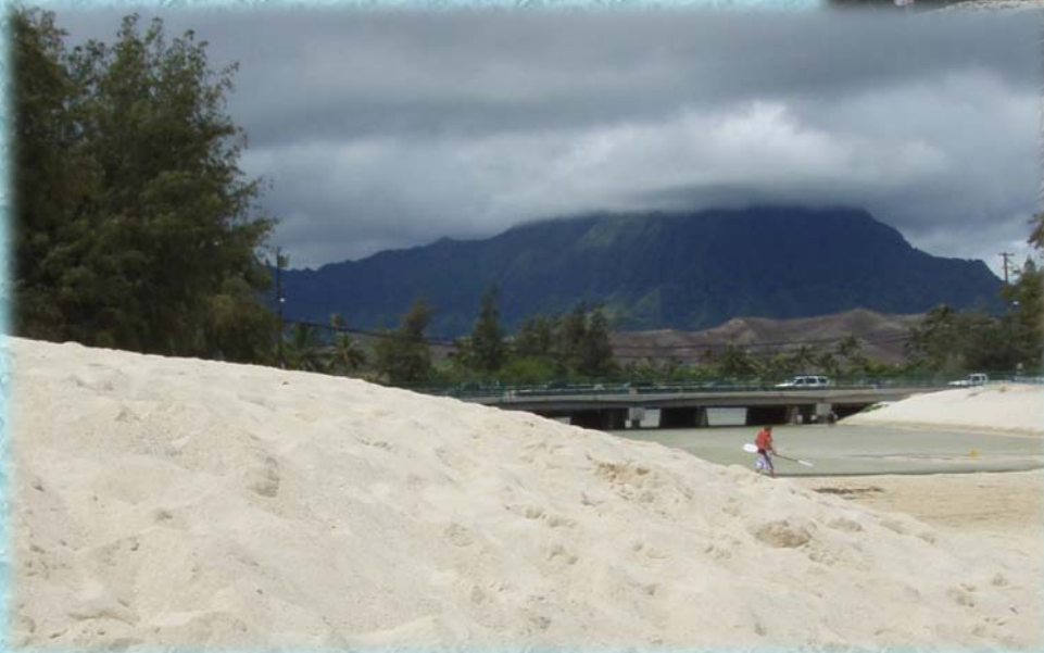
Stream Plugged with Sand
