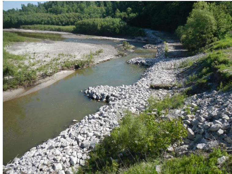
Figure 1. Typical Section 14 Bank Stabilization Project.
