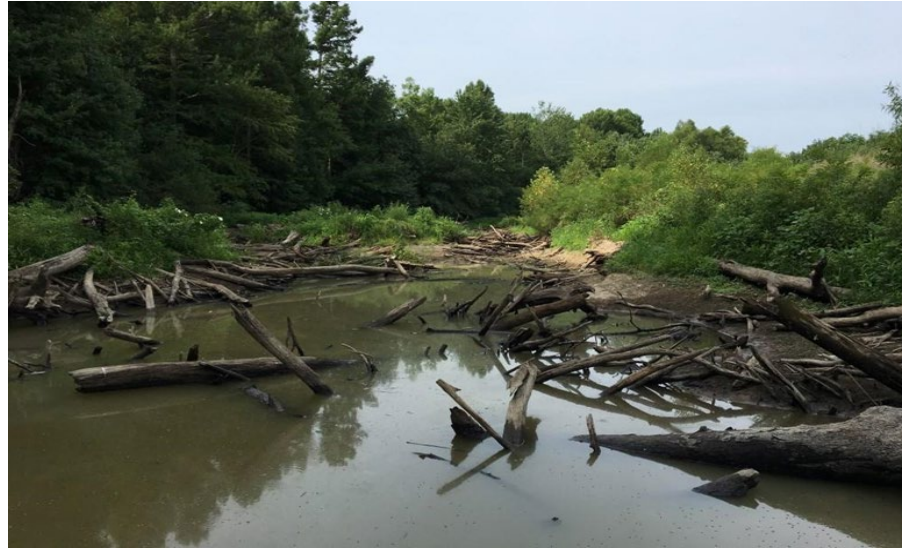
Debris and sediment blockage Below Hwy. 90
