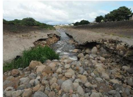
Figure 2: Debris Basin, filled with sediment (left) and scour in the natural leveed reach (right) after the same event (Sep, 2016).
