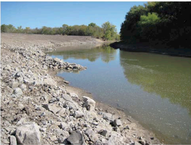
Figure 6. Erosional hotspot upstream of Tuttle Creek Lake before (above) and after (below) stabilization.
