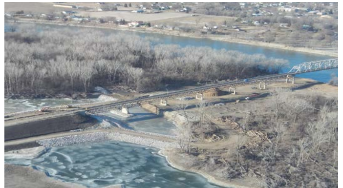
Figure 2. Bridge Abutment Repair at Decatur Bridge
