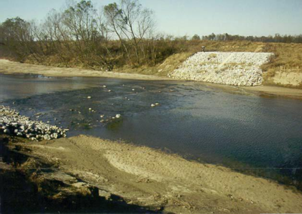
Grade control sills, immediately after construction
