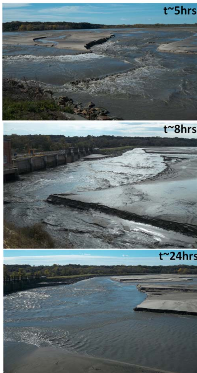
Figure 3. Evolution of the Spencer Reservoir sediment delta during the flush. The head cut propagated upstream shortly after the flushing gate was opened (top). Then the channel deepened and widened the rest of the first day (middle), until it settled into a form close to the final geometry 24 hours after the flush (bottom).
