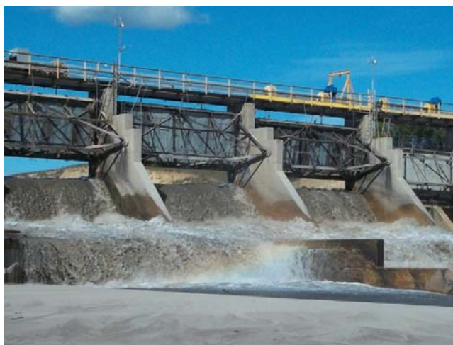
Figure 2: Sediment laden water flowing over the main gates early in the Spencer Dam flush.
