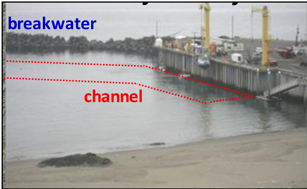
Figure 6. Harbor channel near dock at Port Orford, Oregon, which must be maintained by dredging. Photo shows vessel haul-out along dock face and damaged breakwater (2014).
