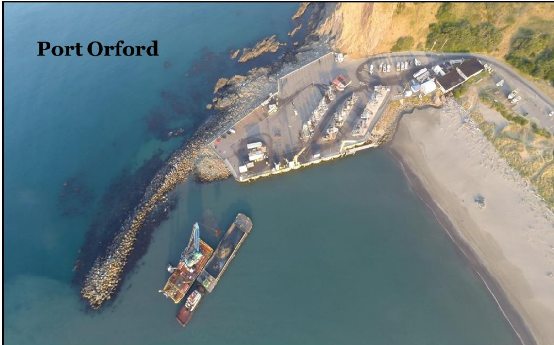
Figure 5. Clam shell bucket dredge and scow dredging entrance channel behind breakwater at Port Orford, Oregon. (photo by City of Port Orford, Oregon.)
