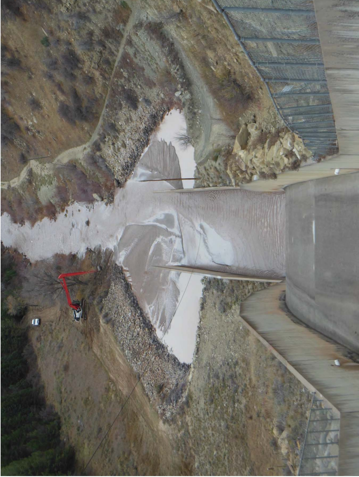
Figure 3- Sediment accumulation downstream of stilling basin observed in 2014.
