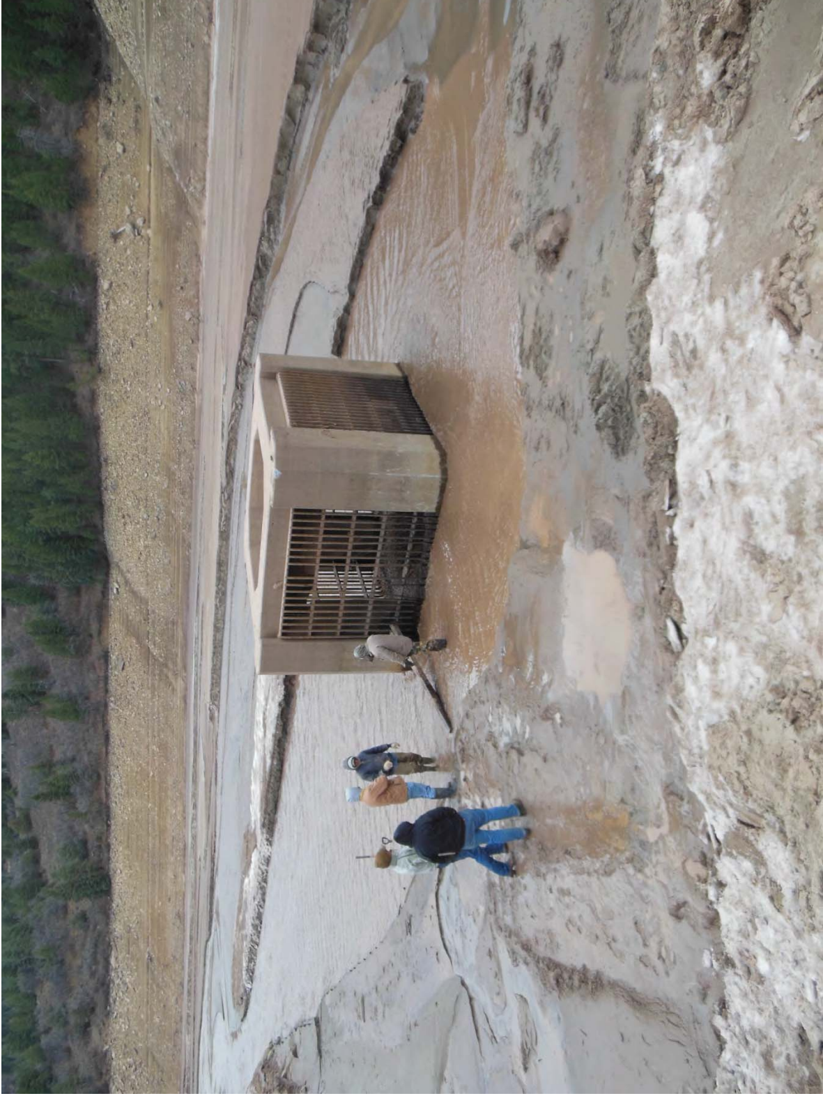
Figure 2- Low flow channel eroded through sediment deposit in 2014.
