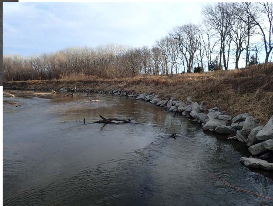
Effective Bank Stabilization Project Longitudinal Stone Toe Protection
