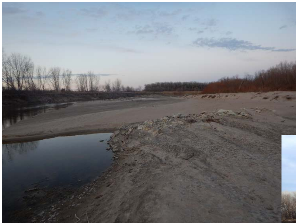
Ineffective Bank Stabilization Project Bend Way Weirs (Flanked)
