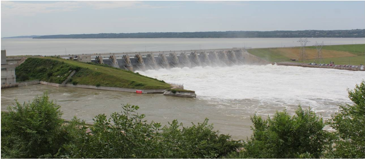
Figure 2. Gavin's Point Dam Discharging 4530 cms from Spillway Gates
